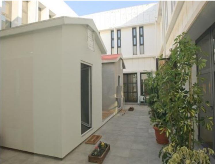
NO degradation using Gypsum board panels with Calcareous TCM1 PC powder
